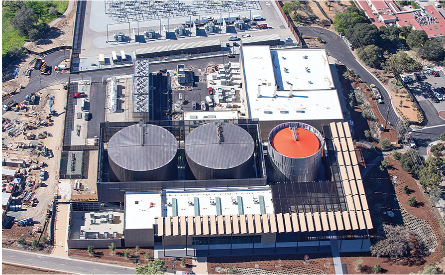
Figure 6.1: The new Stanford campus central plant constructed as part of the $485-million Stanford Energy System Innovations (SESI) project [9]
