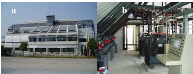
Fig. 15. (a) Shanghai Green Building; (b) adsorption chiller powered by solar energy.
