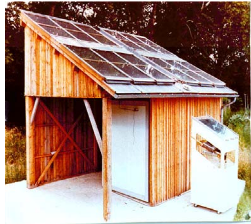
Fig. 9. Cold storage room.
